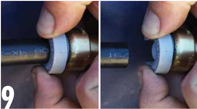
Grasp the fitting and the removal sleeve in one hand, pulling the sleeve toward the fitting. The pipe should pull away easily with the other hand.
