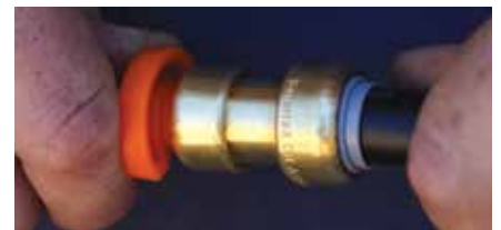
Once again, it is crucial to cut tubing squarely and without a burr. The small tube cutter (about $20) is perfect for the task.
