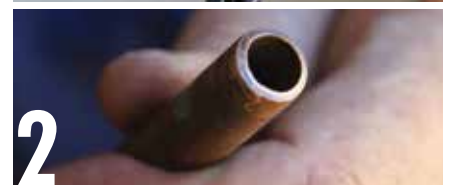
Once again, it is crucial to cut tubing squarely and without a burr. The small tube cutter (about $20) is perfect for the task.
