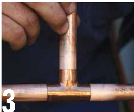
3 Fit the pipes into the socket, making sure they extend into the sockets to maximum depth. There is no need to apply any flux to the joint for copper-to-copper joins.
