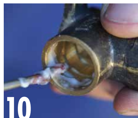
10 To join copper pipe to a brass fitting, coat the inside of the fitting with water-soluble flux paste. You may also apply flux to the tip of the pipe.
