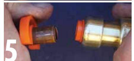
Removing a fitting is the same as for PEX pipe, provided you have the correct sized orange removal tool for copper pipe.
