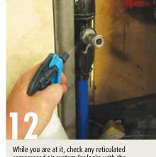
compressed air system for leaks with the detergent mixture. The air compressor will cut in continually to maintain the system pressure if there are even small leaks. If you tend to leave the system on, this will cost electricity.
